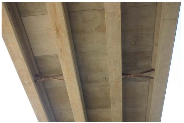
NOTE: Two temporary timber construction x-braces remain in the 2nd span from the North over the creek channel.
