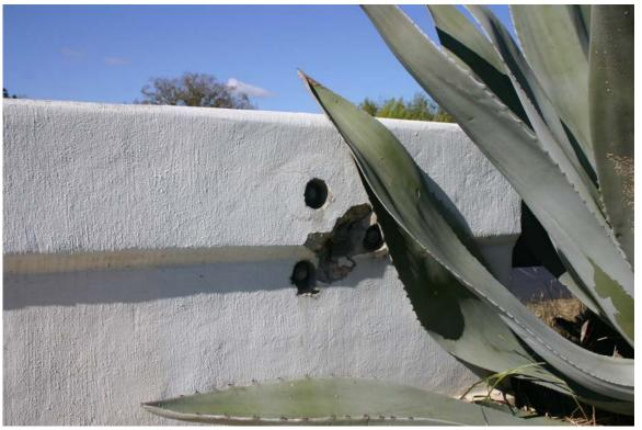
NOTE: A few very minor spalls in the outside face of the concrete bridge rail at the NE approach guardfence bolted rail transition connection.
