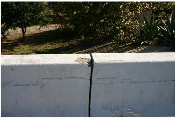
NOTE: Very minor shallow cosmetic spall in the top of the concrete bridge rail at the SE bridge corner.
